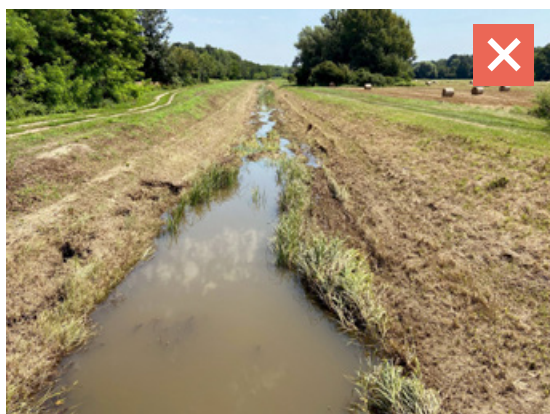
↑ FIGURE 4.2.10 An example of poor practice: vegetation growing along the watercourse mown with a mulcher, at some places even all the way to the ground (location: Gliboki Stream) (Author: Martina Šašić Kljajo)
