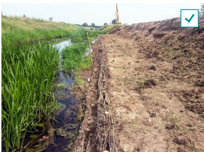
↑ FIGURE 4.2.40 An example of good practice in implementing bioengineering methods to stabilise a slope of a small watercourse at a site in Međimurje; using fascines to stabilise the slope (↔ left); at a site in Nespeš, Sv. Ivan Zelina; using fir tree boards and stakes to stabilise the slope (↔ right) (Source: Croatian Waters)
