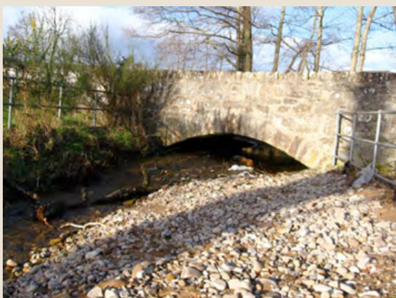
← FIGURE 4.2.7 An example of the implementation of Measure A.2.: sediment is removed only if and where necessary, i.e. where it obstructs the flow and thus presents the risk of harm to the health and property of people; sediment deposits found next to a bridge may increase the risk of flooding (Source: Scottish Environment Protection Agency 2010)
