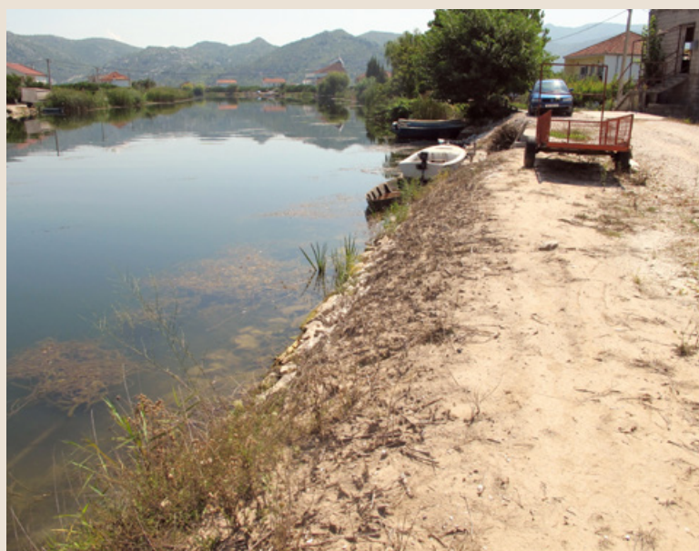
↑ FIGURE 4.2.42 A new earthfill revetment (location: Mala Neretva) (Source: Institute for Environment and Nature, MESD)
