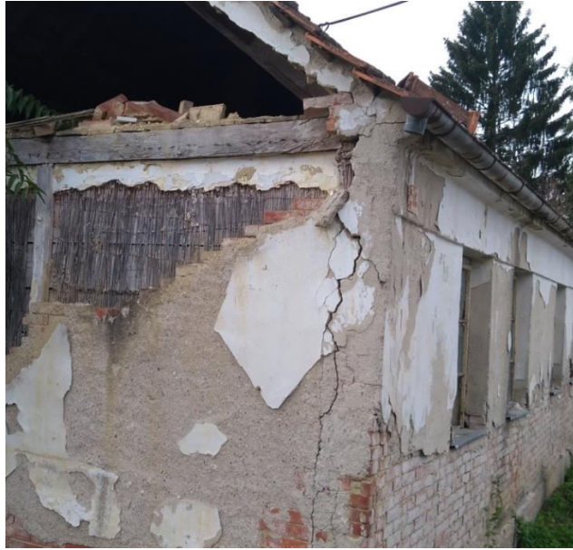
Figure 3: Example of using reed as an insulation material in old houses in Zlatar
