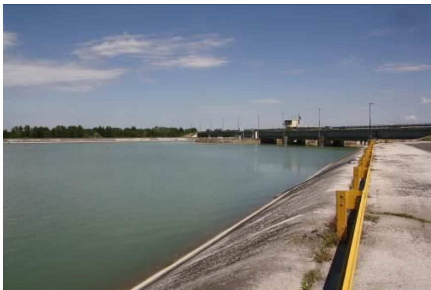
Figure 31: Čakovec reservoir dam with the outlet to the derivation canal (right), and the old Drava river bed (left).
