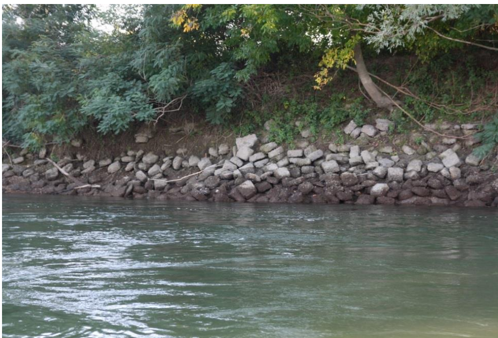
Figure 15: River banks protected by rip-rap structures
