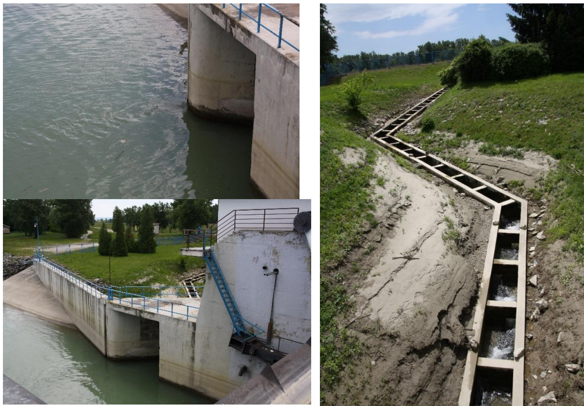
Figure 32: Fish passage at the Čakovec reservoir. Weak current at the inlet may not attract fish sufficiently to enter the passage. High slope (right) results in low efficiency of this device.
